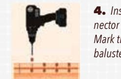
**4.** Insert a screw through the baluster connector and install where the lines intersect. Mark the center for placement before installing baluster connector.
